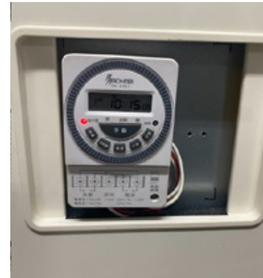
▲ Installed timers on air conditioning units to ensure they are powered off after working hours and during holidays.
